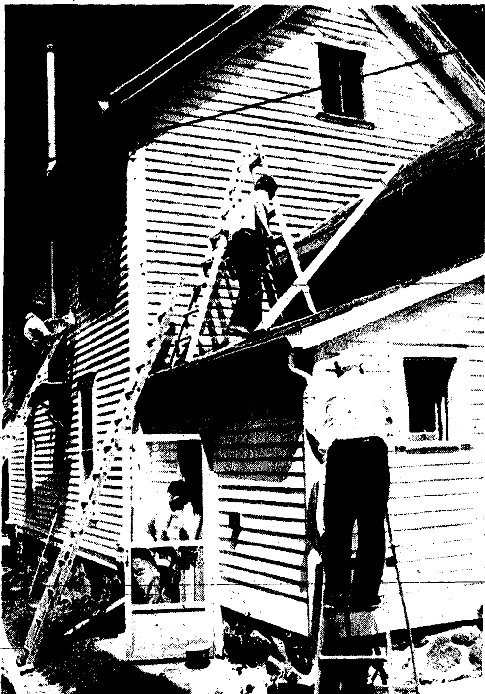
CHRISTMAS IN APRIL program has extended into June in Chelsea. Lions Club members worked last Saturday to finish painting a Congdon St. home in the program. The program, held county-wide for the first time, helps rehabilitate homes for elderly, handicapped, or low income homeowners. It is completed entirely by volunteer labor and donations. In the door is David Jaehalke, on the roof is John Groesser, on the step ladder is Roy Clemons, and on the extension ladder is Lary Bailey.
