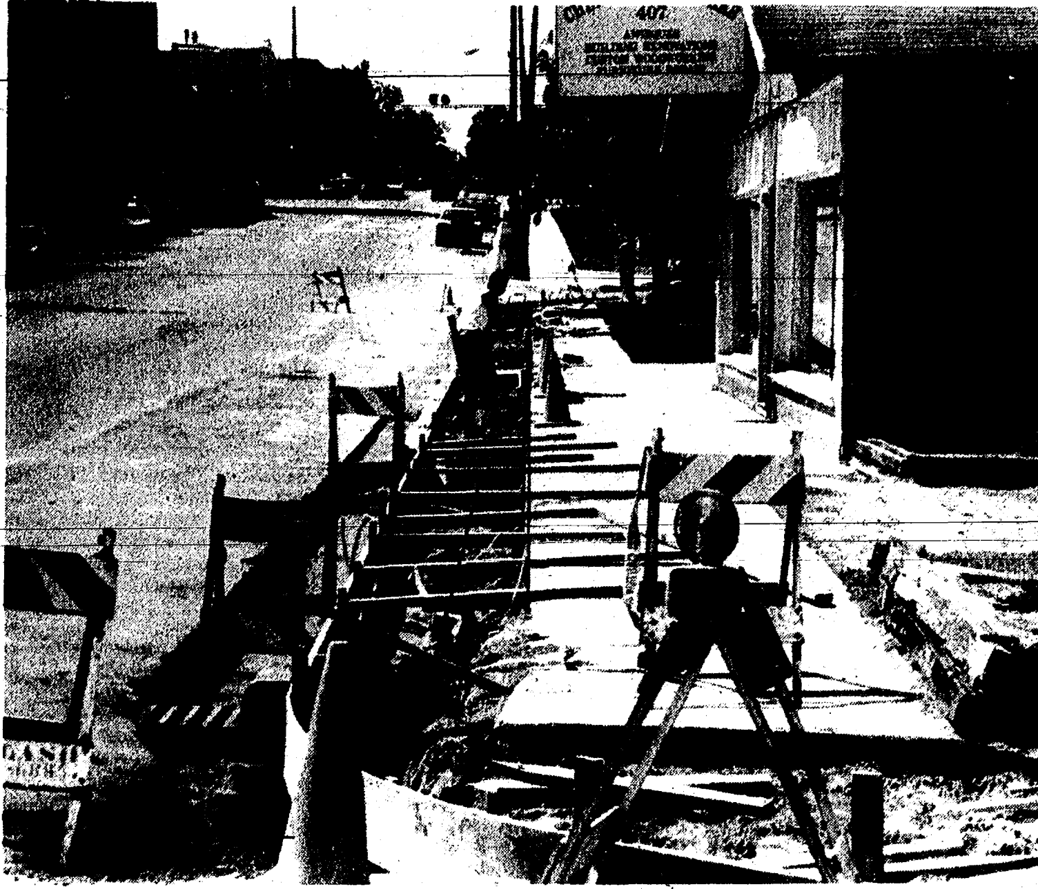
FINAL PORTION of the downtown streetscape project is being completed on N. Main St. this week. Contractors are scheduled to have most of their equipment and supplies out of town by the end of the week.
